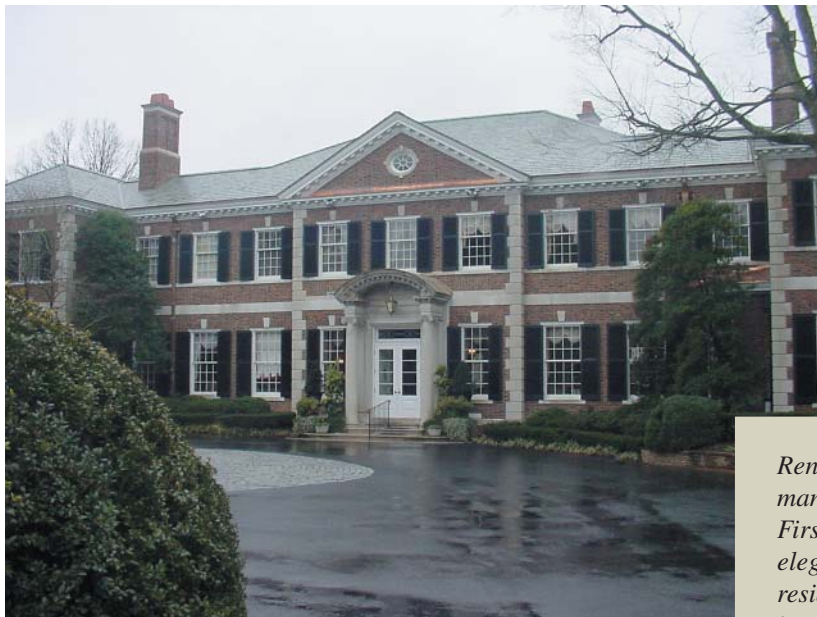
Courtesy of Nashville Electric Service.
