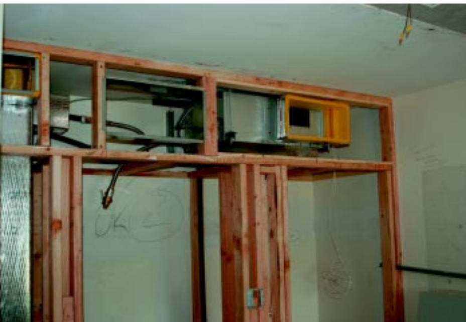
The units were installed in these spaces above the closets in the women's rooms.
